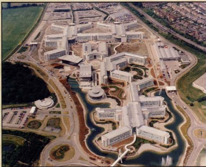
▲ Ministry of Defence headquarters at Bristol. One of the latest in a long line of major Audix projects, linking eleven buildings over complex audio and data cable networks and providing comprehensive voice alarm and public address communication in all areas.
