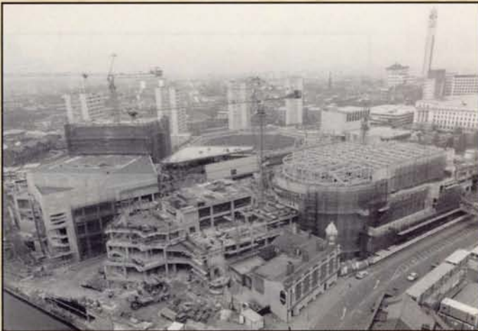
▲ ICCB under construction alongside the NIAS in the heart of Birmingham.
